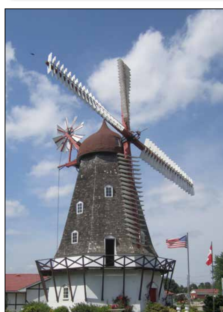
This Danish smock mill, originally built in 1842, was taken apart and re-assembled in Elk Horn, Iowa, in the 1980s. It is an advanced type of mill; notice the lowered sails that can be easily controlled from the deck at the bottom of the mill. Also there is a wind vane at the back that turns a gear to hold the sails steadily into the wind.
